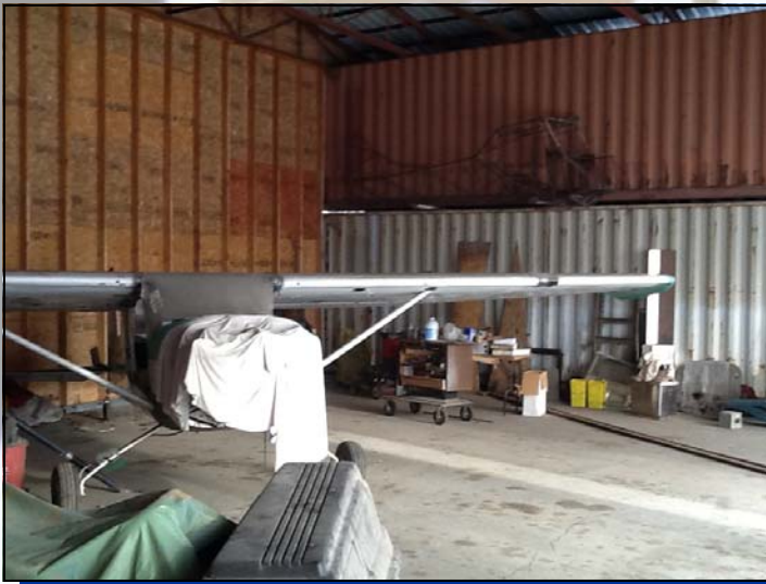
Interior of the main hangar bay facing Northeast. The airplane is Syd's. About 18 ft from the bottom of the trusses to the hangar floor.
